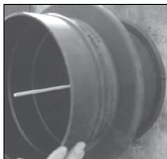
Place the sleeve over the end cap nailed to the form.
