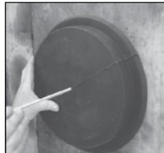
After nailing end cap to form, drive (threaded rod\*) through the end plate and form and (thread nut\*) on other side.
