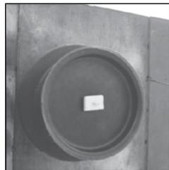
Place second cap on the sleeve and use a (block of wood\*) and (wing nut\*) to tighten unit in place. Make certain sleeve is plumb.
