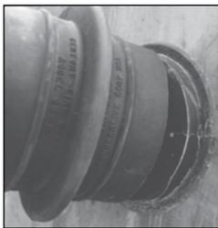
3. Place the Century-Line® Sleeve on the end cap. When field cutting non standard CS sleeve lengths, the sleeve and end caps total length should be ¼" longer than the thickness of the wall. Cut with a hand or power saw.
