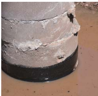
Riser-Wrap® used to rehab. an existing manhole submerged in runoff water.
