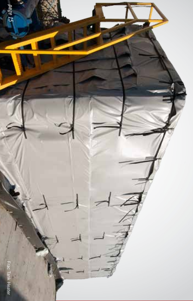
Silo Tank Heating Blanket
