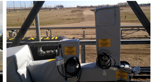
TOP: Freeze protected piping MIDDLE LEFT: Freeze protected truck mounted propane tank MIDDLE RIGHT: Freeze protected CID2 safety shower BOTTOM: Aircraft engine preheater
